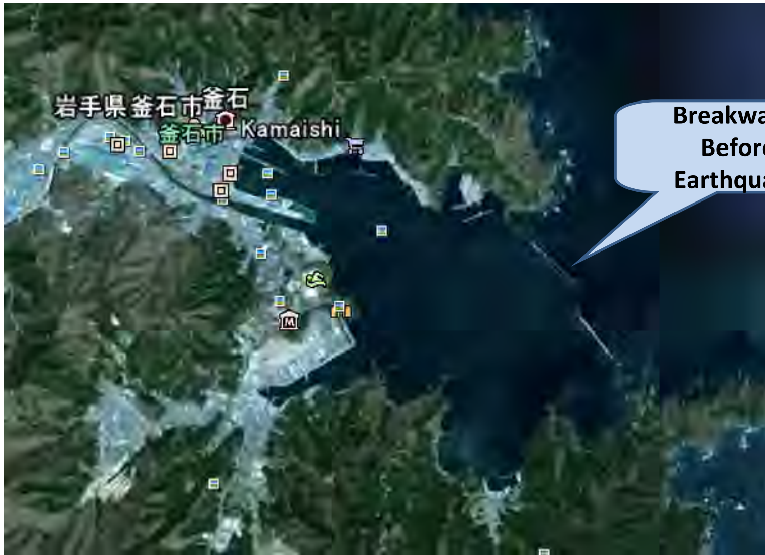
Fig.4a The Deepest Breakwater against Tsunami in Kamaishi Bay. Iwate Prefecture
