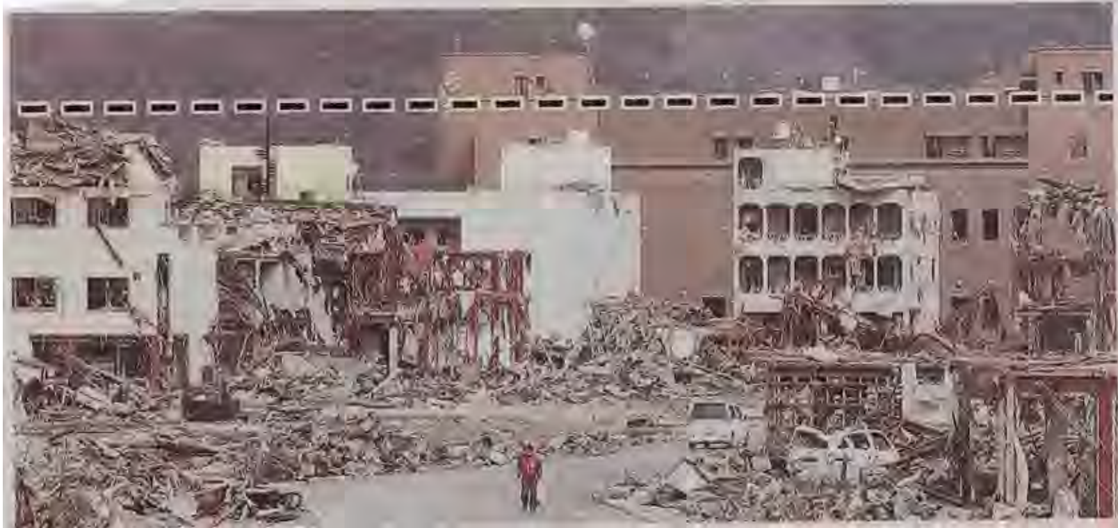
Fig.6 Water Level of Tsunami (15m) in Onagawa Town Up to the Roof of the Fifth Floor Building
